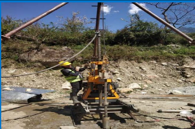
Monitoring SPT test at Powerhouse, USHEP
