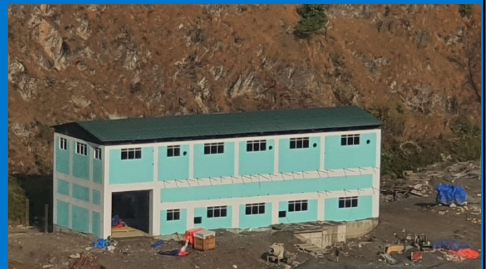
We assist implementing the design (15.33MW) KGHEP PH under construction)
